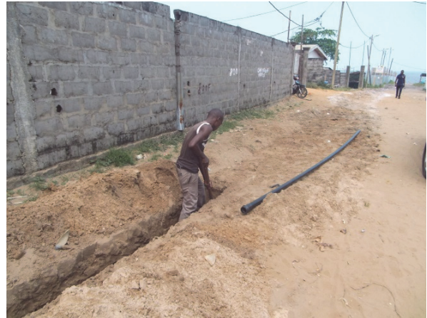
Construction of water supply facilities by Congo government (2014.6)
