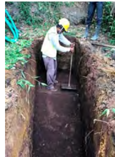
Tamping by steel tamper (~ 10kg) for compaction and smooth finishing.
