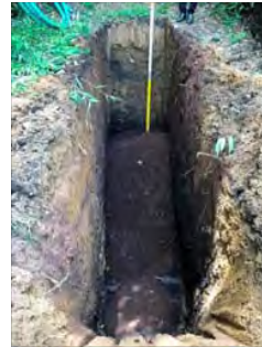
PRB filling on third layer (~0.5m)
