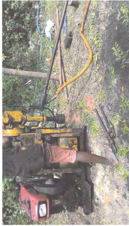
Fig. 10 - Machine setup for drilling at BH-05
