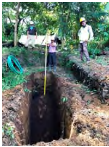
Filling the forth layer (0.5m).
