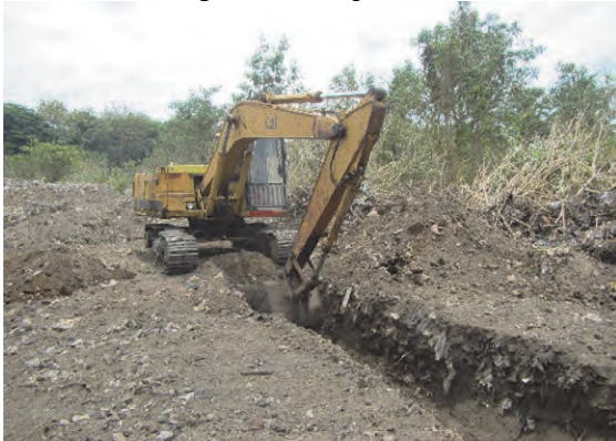
Demonstration of PRB construction
