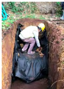
Laying the separation geotextile before backfilling with excavated clay soil.
