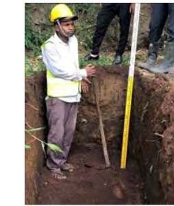
After filling up to final height (124.5m) that is 1.0m below the 125.5m surface level.
