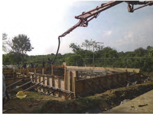
Construction of night soil treatment plant in KPS
