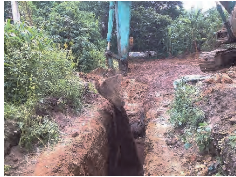
Filling the mixed PRB materials
