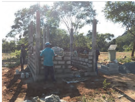
Construction of Block walls
