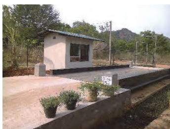
Weigh Bridge System
