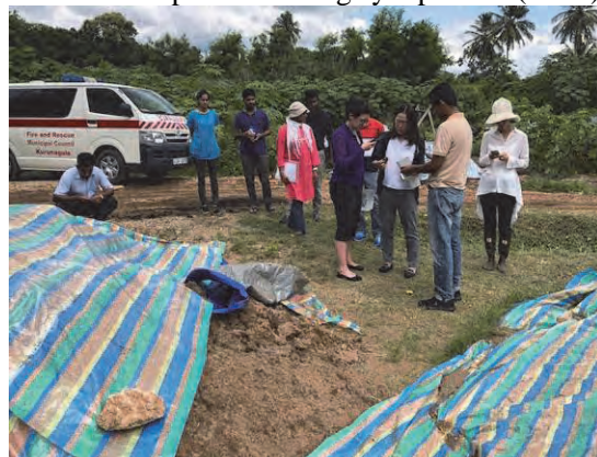
Stocked PRB material at landfill site in KPS
