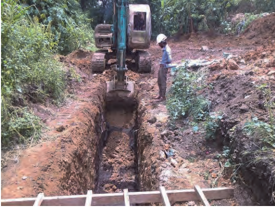
Construction of the PRB at KMC
