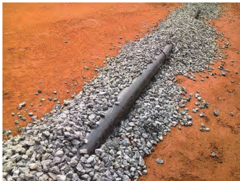
Percolated pipes for branch line is covered by aggregates
