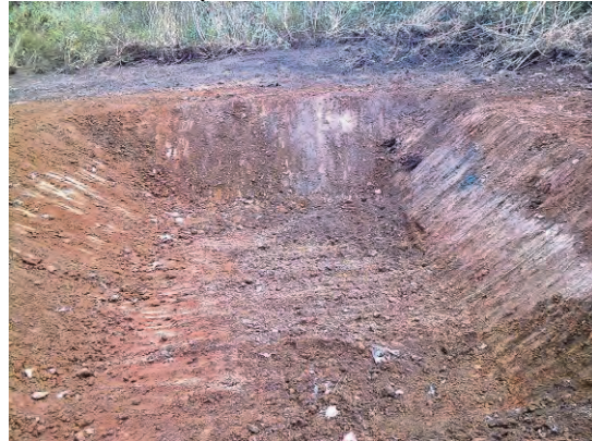
Construction of the working yard
