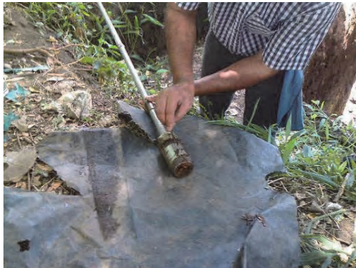
Sampling of the compacted PRB layer
