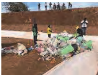
Discharging of residue waste
