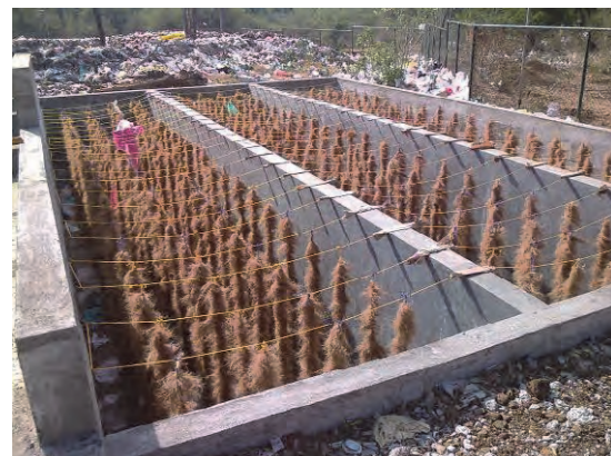
The COTS is installed
