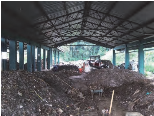
Progress of windrow type-compost production (RMC)
