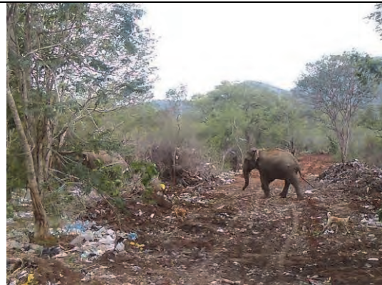
Before installation of the electric fence: elephants appearing during the construction works
