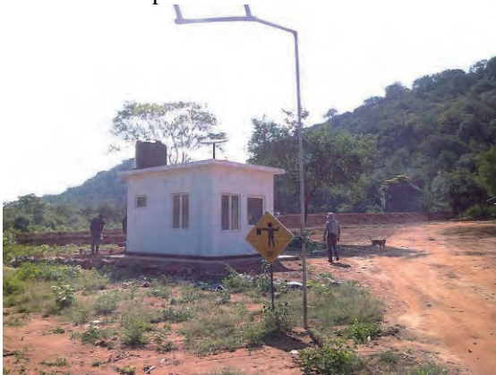
Completion of the Security hut (25th April)
