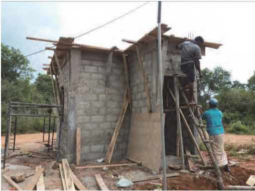
Construction of a Security Hut in the Dumpsite in KPS
