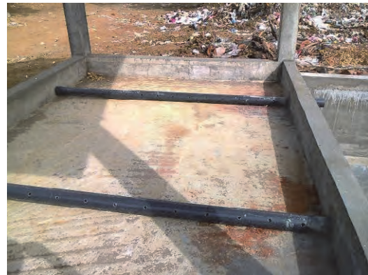
Percolated pipe for the sludge drying bed
