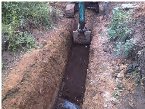
Compaction for the PRB layer Required level of compaction is 1.0-1.1 kg/m 3
