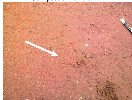
Coconut coir fibers were mixed with the bentonite-soil layers
