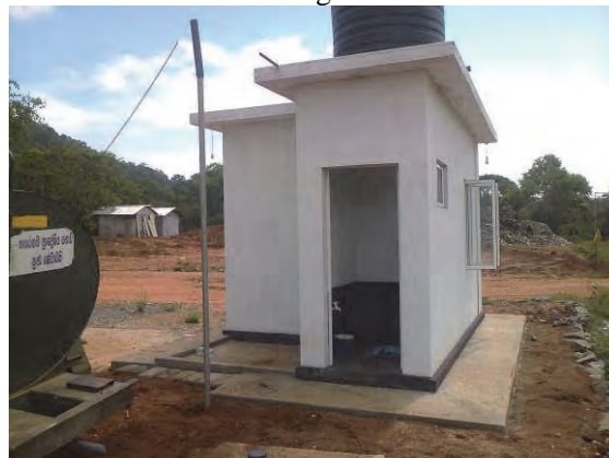
Completion of the security hut (26th April)
