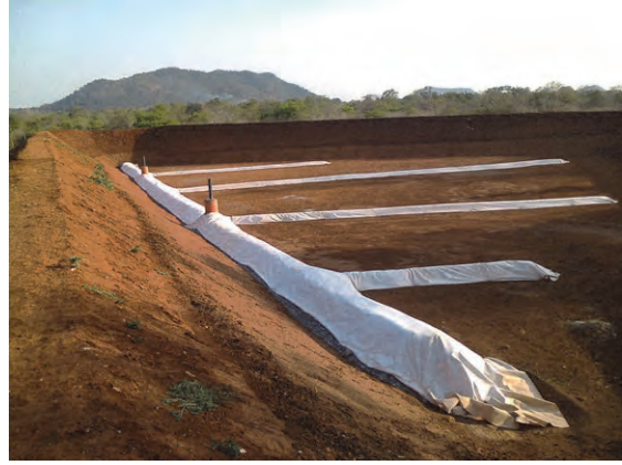
Completion of the construction of landfill site in KPS
