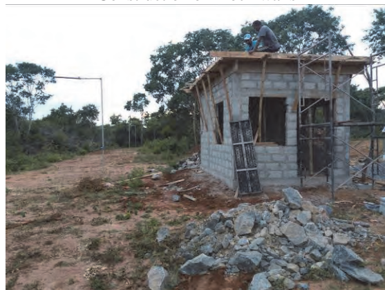
Form working of the roof
