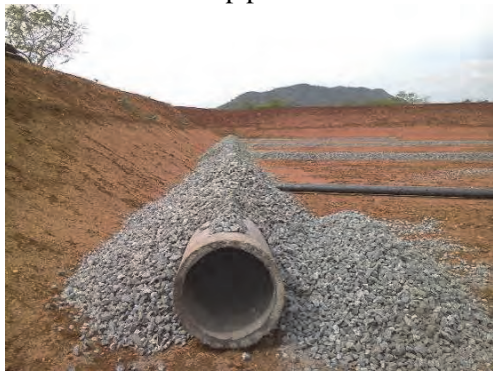
Trunk line pipe
