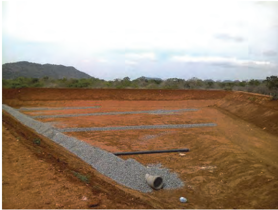
The photo after completion of earth works and leachate pipes were installed (August 2018)
