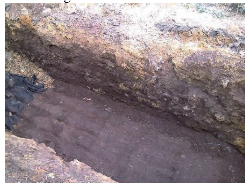
The compacted PRB layer
