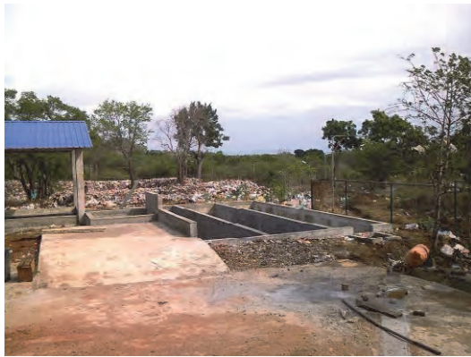
Night soil treatment plant (August, 2018)
