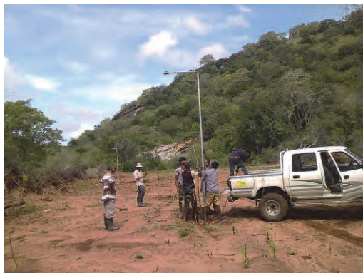
Construction of elephant fence at Galapitigalayaya disposal site (KPS)
