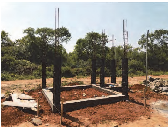
Construction of the Pillars
