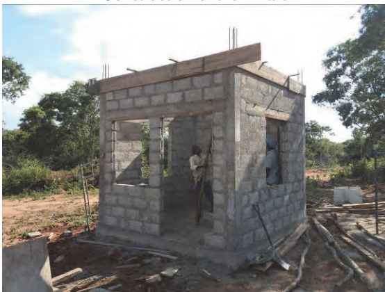
Completion of the Block Walls
