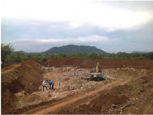
Progress of construction of disposal site in KPS
