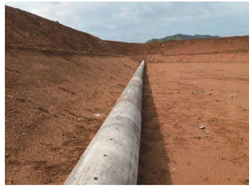
Percolated concrete pipes for the trunk line
