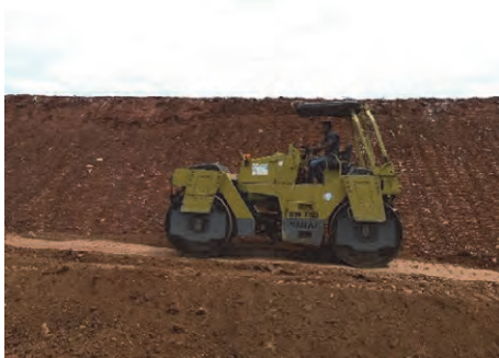
Compaction for the liner
