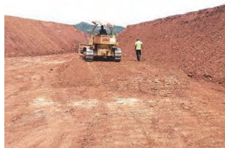
Compaction for the liner
