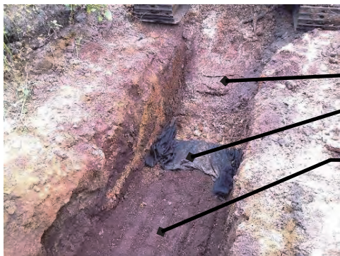
Figure 2-30: The Model of PRB installation
