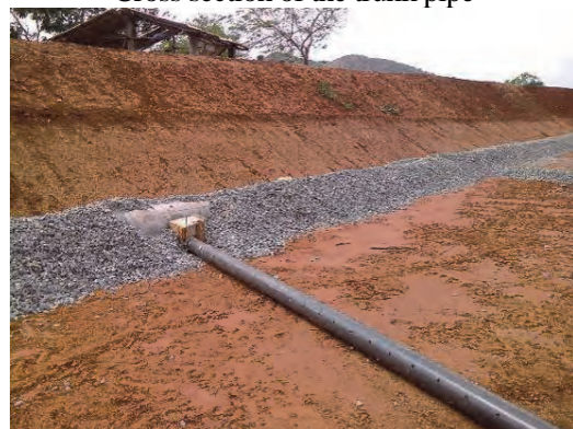
A percolated pipe for the branch line is connected to the trunk line pipe
