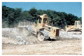
Figure 8.1.1 Wastes compacted by bulldozer/compactors
