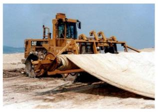
Figure 2.4.1 Application of Geotextile Matting
