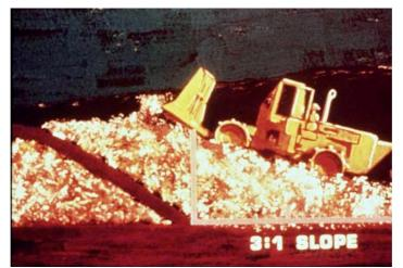
3H:IV-as shown at Figure 8.2.1) to maximize the compaction effort of the machine.
