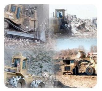
Figure 7.2.1 Placement of the first layer of waste
