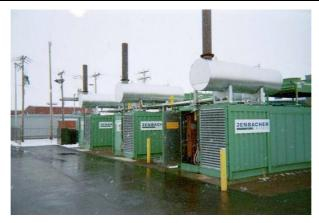
Figure 14.6.1 Gas engines
