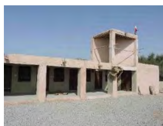
Guest service facilities
