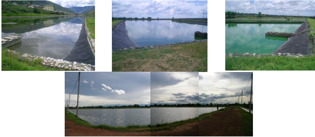
Note: Top left: Thimphu STP in Bhutan, middle/right: Phuentsholing STP in Bhutan, bottom: Kamphangphet STP in Thailand Source: JICA Project Team
