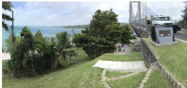
Figure 10-3-2-1.2 Situation around the hand hole adjacent to KB bridge
