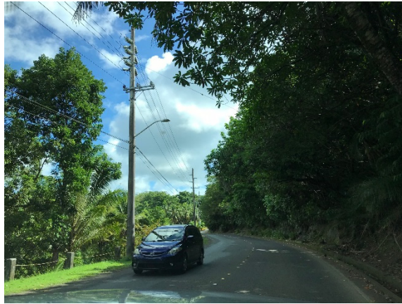
Figure 10-3-2-1.3 A place where it will be difficult to secure the space necessary for new pole installation (example) (Near the entrance of Koror downtown)
