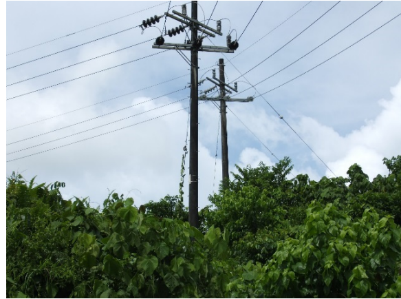
(b) Example of a vine climbing up a guy wire
