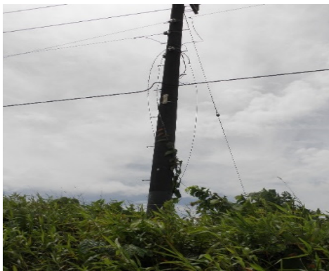
Figure 9-1-4-1.7 A vine guard preventing growth
