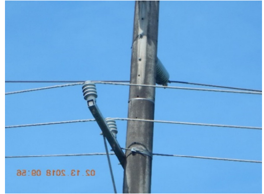
Figure 9-1-5-1.3 Inclination of the arm
