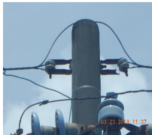
(b) Broken support hardware for the insulator by rust
