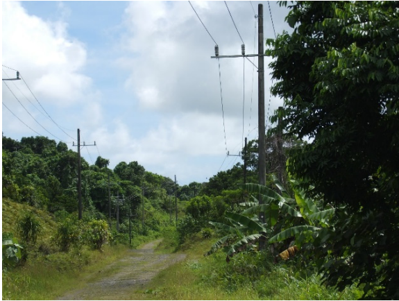
(a) Vine guard installation on the Nekken T/L
