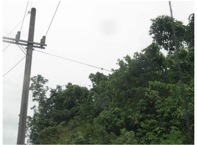
(b) Winding around a guy wire
