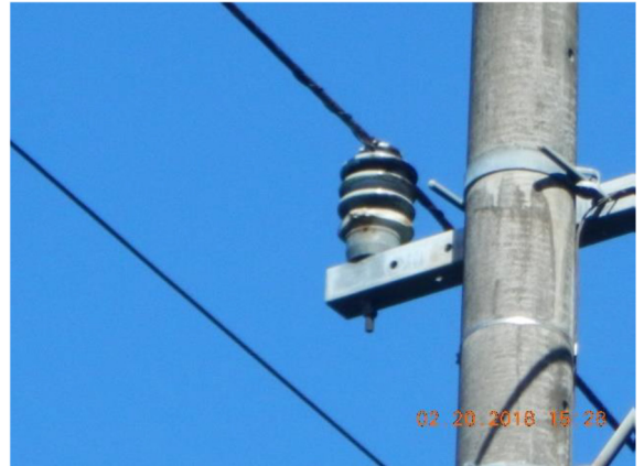
Figure 9-1-5-1.5 Chipped insulation
