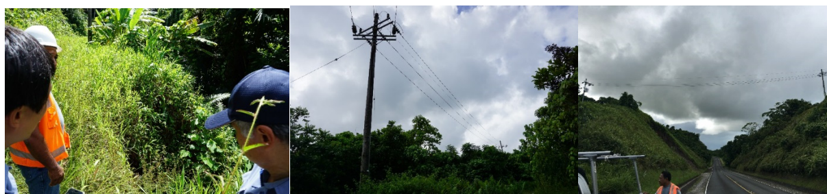
Landslide along the old road line running over the trees line running on the hills
