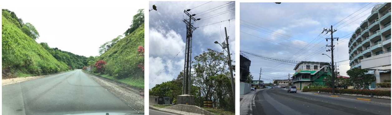
COMPACT Road Existing cable-pulling pole near KB Bridge Downtown Koror
