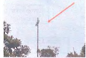
Difficult to find the condition in fault patrol
