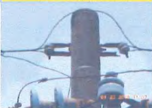
Breakage of clevis found by patrol
