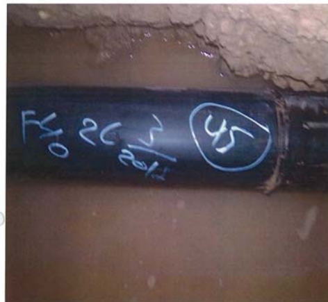
Joint # 45 Location IP3 +720' Straight Date 26-Mar
