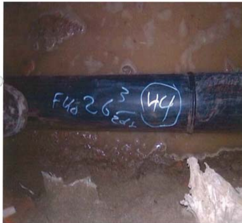
Joint # 44 Location IP3 +680' Straight Date 26-Mar
