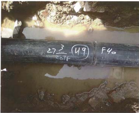
Joint # 49 Location IP3 +877' Straight Date 27-Mar
