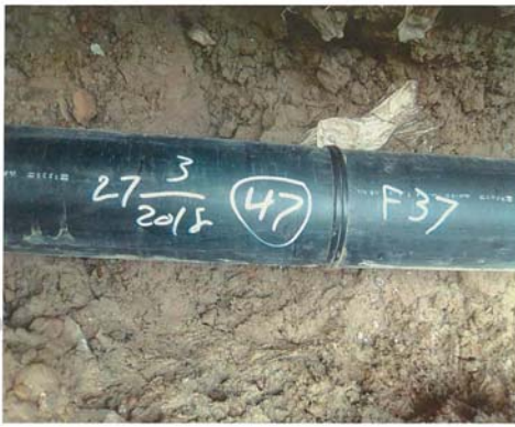
Joint # 47 Location IP3 +800' Straight Date 27-Mar
