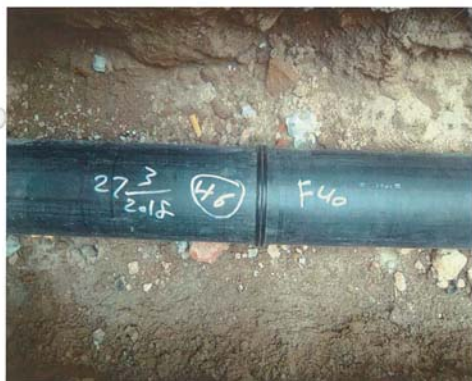
Joint # 46 Location IP3 +760' Straight Date 27-Mar
