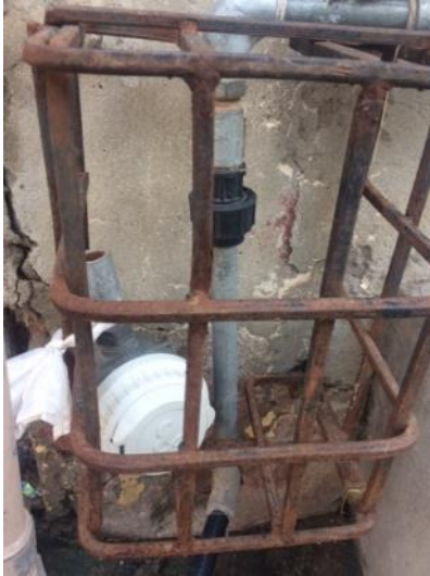
Removed stuck meter
