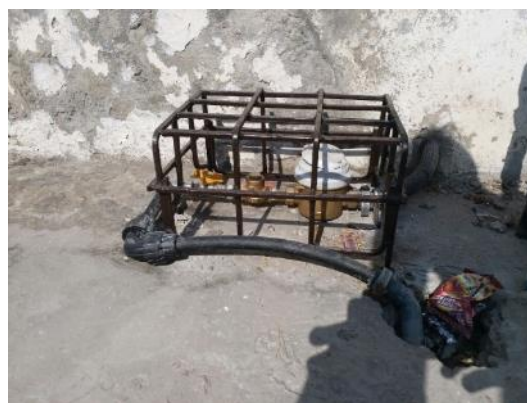
Narrow space connection
