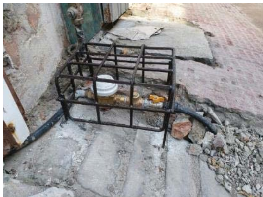
Connection on a slope
