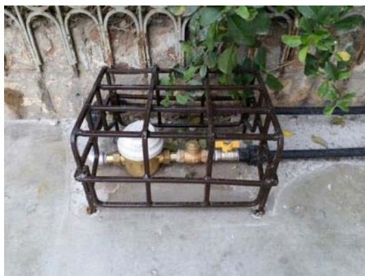
Meter installation (on the surface)
