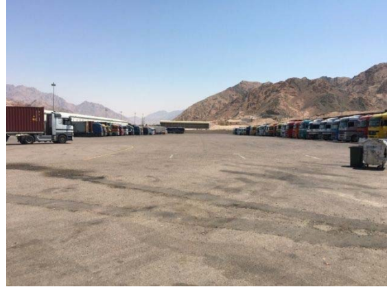
Manual inspection site at Yard-4 (more than 80 inspection booths)
