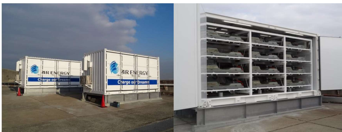
Photo 9-1 Reuse Battery: (left) Exterior, (right) Inside of package
