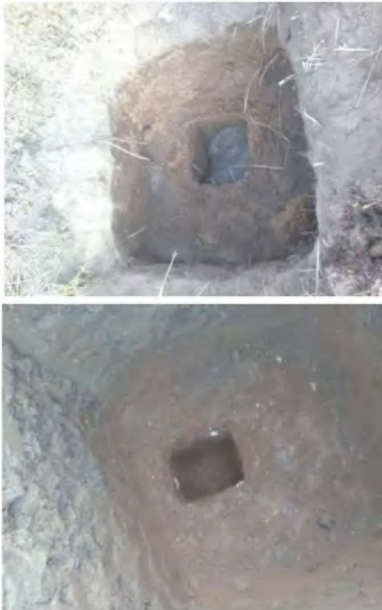
Figure 10. Test pit opened for the percolation test (left) and pre-soaked pit for the percolation test.
