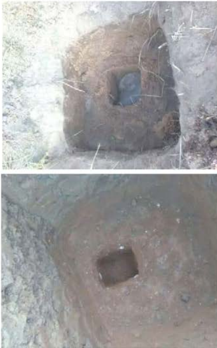
Figure 10. Test pit opened for the percolation test (left) and pre-soaked pit for the percolation test.
