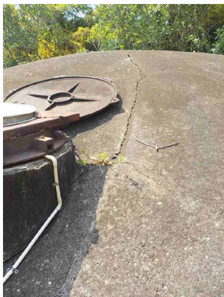
Photo 2.2.2 Conditions of cracks on the top of the Phousi Reservoir
