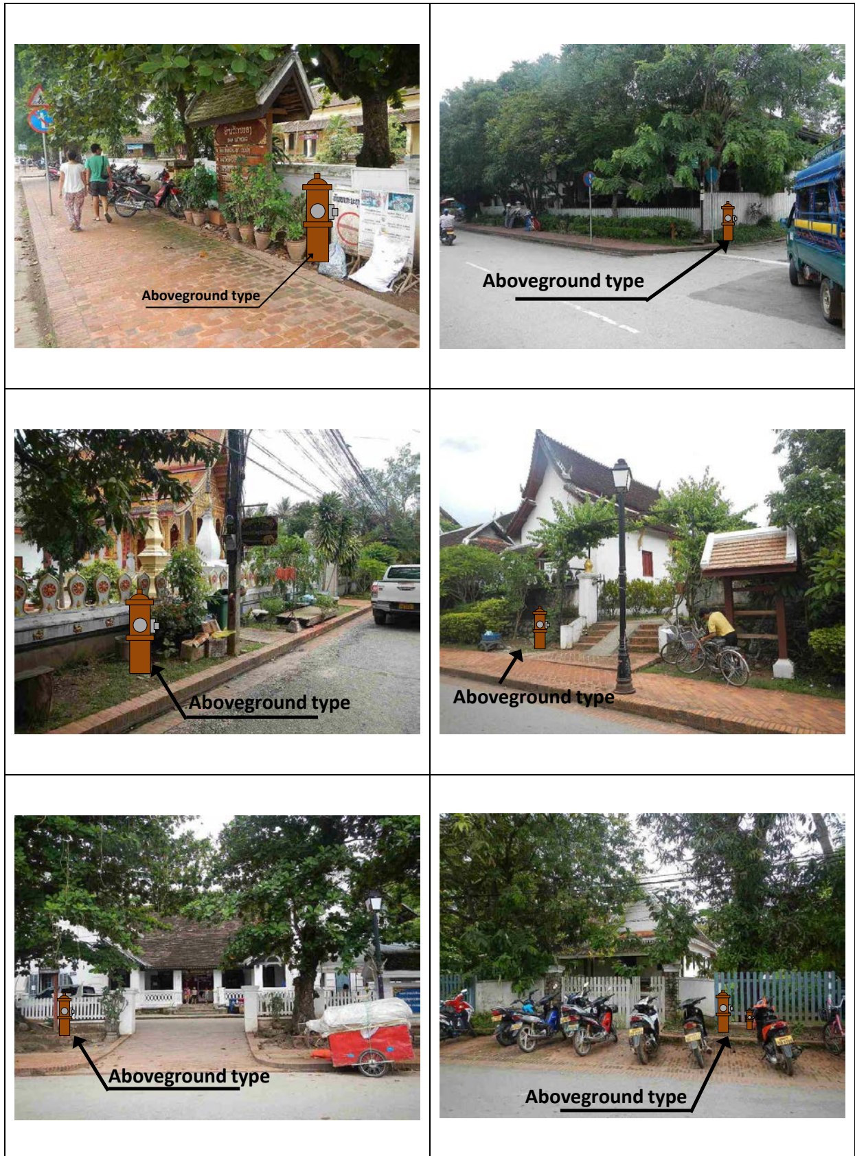
Photo 2.2.6 Installation of fire hydrants above ground
