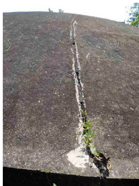
Photo 2.2.2 Conditions of cracks on the top of the Phousi Reservoir
