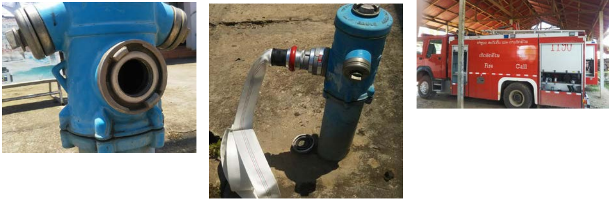
Photo 2.2.5 Coupling on existing fire hydrants
