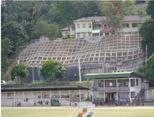
Figure 3.2 Entire view upon completion
