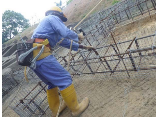
Figure 3.3 Frame assembly
