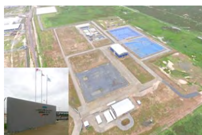
Overview of Treatment Facilities
