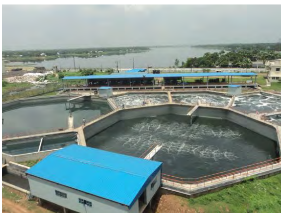
CETP at Dhaka EPZ (Owned and Operated by
