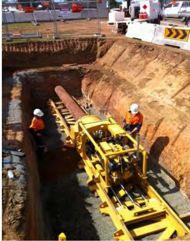
Figure 3.3-5: sample image of thrust boring for road crossing
