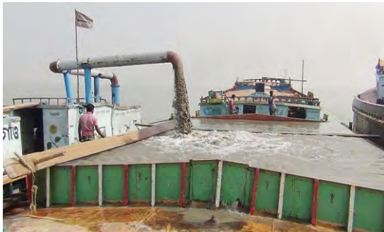
Dredging of fill material from the river bed at Meghna river by pumping up
