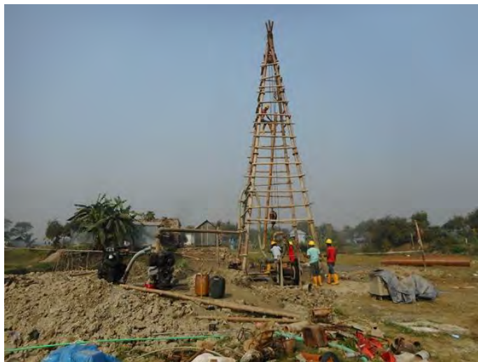
Figure 2.2-6: Photograph of drilling site at TW-2
