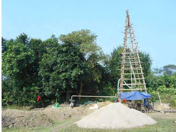
Figure 2.2-5: Photograph of drilling site at TW-1
