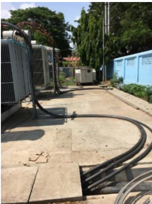
Figure 4.2-1 Secondary cables in a substation laid directly on the ground and exposed to exterior
