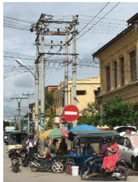
Figure 6.3-2 Distribution line design using 4 concrete poles (in Mandalay City)
