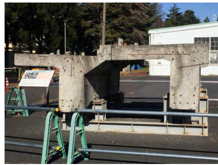
7) Outdoor exhibition area (Sample of RCT beam section)
