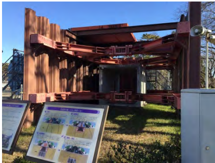
9) Outdoor exhibition area (Construction process introduction area)
