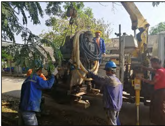
Photo - 1.1 Mobilization of Equipment
