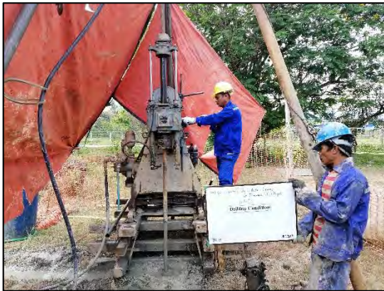
Photo - 1.3 One of drilling condition
