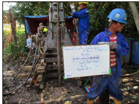
Photo - 3.8 Taking Undisturbed Sampling
