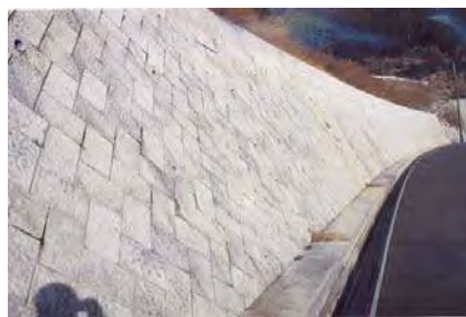
(Concrete block retaining wall)
