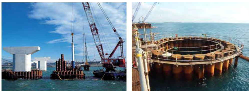
Figure 6.1.6 Image of SPSP (Steel Pipe Sheet Piles) Methodology
