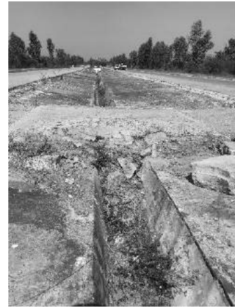
Damaged Drainage
