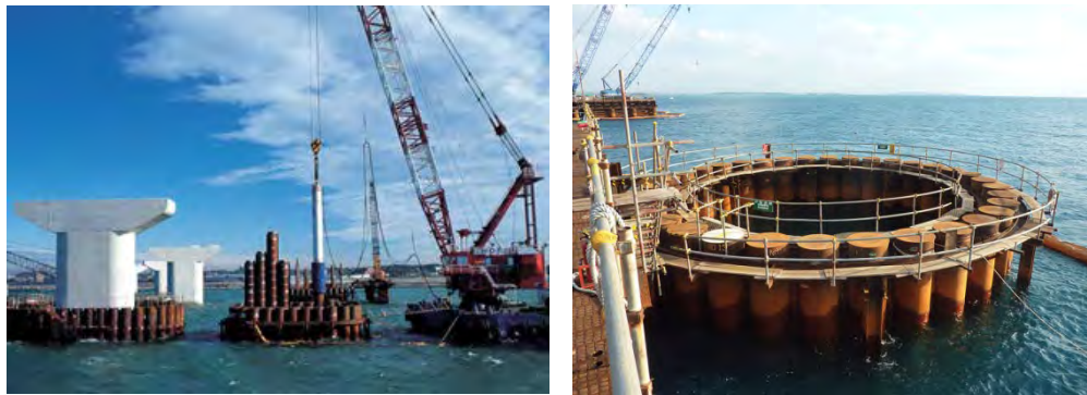
Figure 11.7.6 Image of SPSP (Steel Pipe Sheet Piles) Methodology
