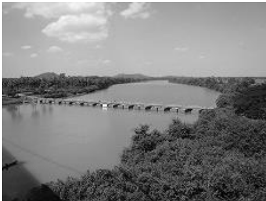
Photo-13 Pontoon Bridge
