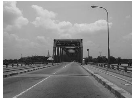
Photo-7 Road Condition on Existing Sittaung Bridge
