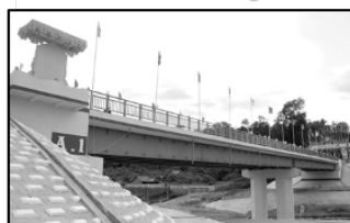
Steel Plate Girder Bridge
