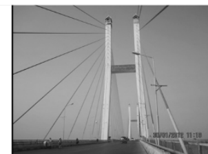
Cable Stayed Bridge
