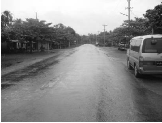
Photo-10 Road Condition on Thaton – Eindu Section
