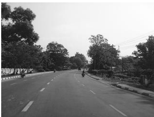
Photo-3 Road Condition on Bago–Payagyi Section
