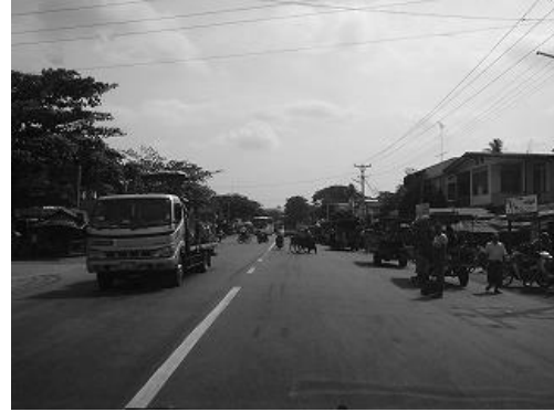
Photo-5 Road Condition at Waw
