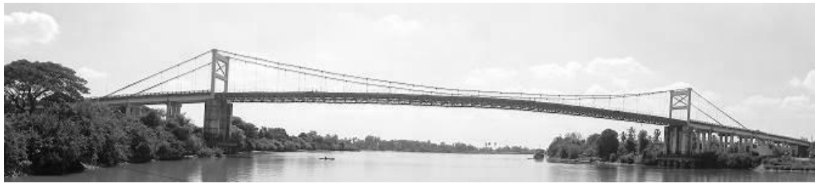
Photo-12 Gyaing Kawkareik Bridge (Existing)
