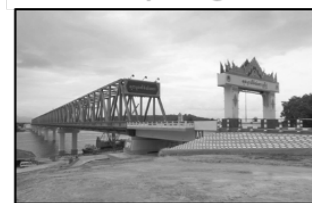
Steel Truss Bridge
