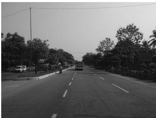
Photo-1 Road Condition on Yangon – Bago Section
