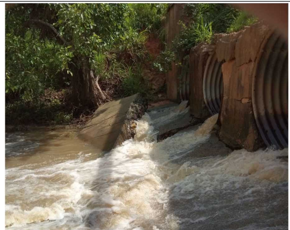
Deformation of river bed at outlet of downstream side
