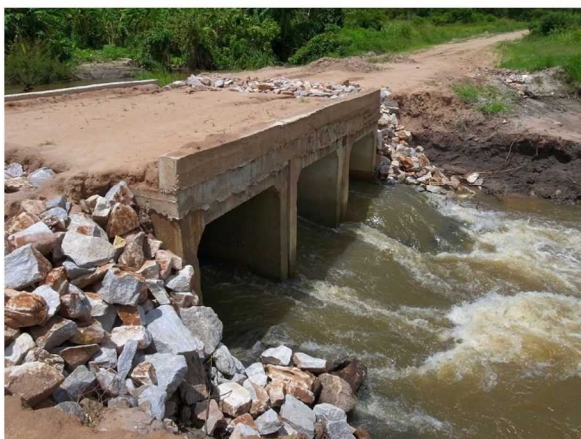
Box culvert on the detour (currently not allowed due to erosion)
