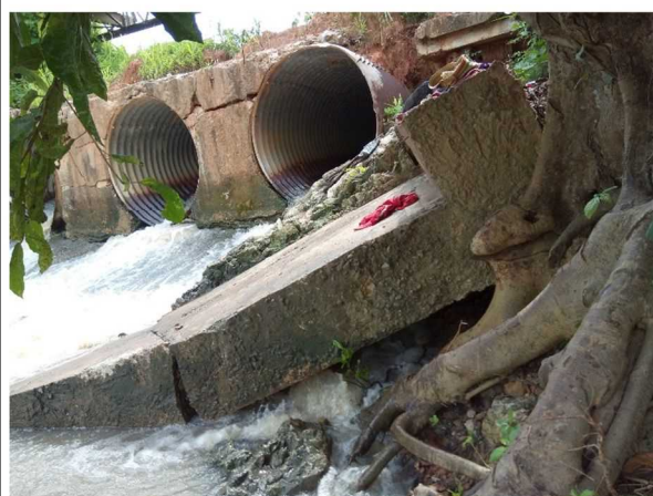
Damage of existing pipe culvert
