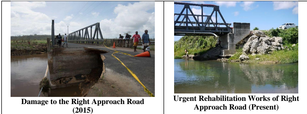
Figure 2.1-10 Teouma Bridge Damaged by Cyclone Pam
