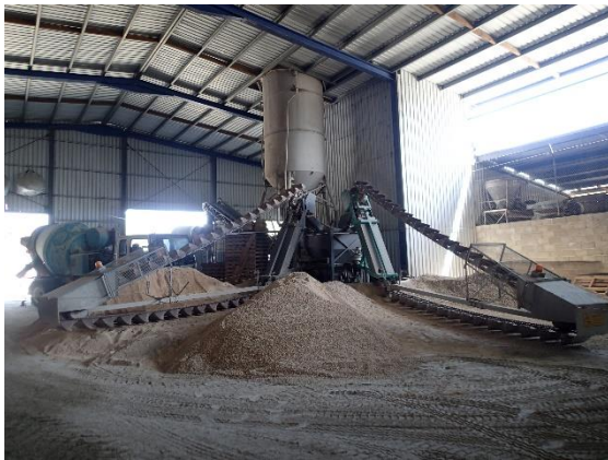
Ready-mixed Concrete plant
