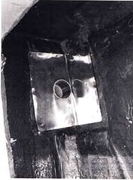
C. REDRAIN INSTALLED DETAIL
