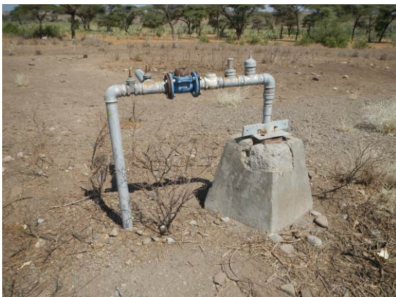
Figure 1-14 Test well
