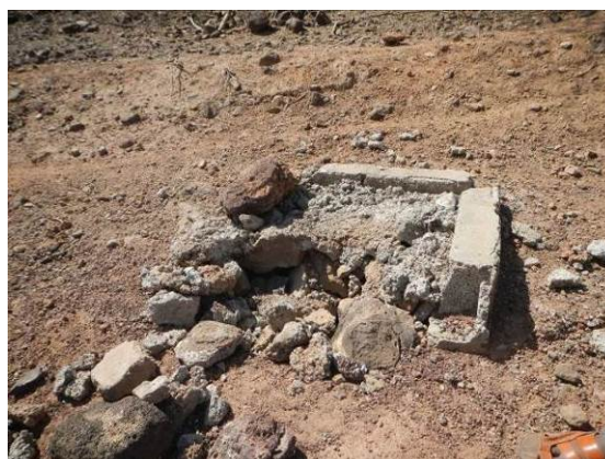
Figure 1-53 Chamber of air release valve
