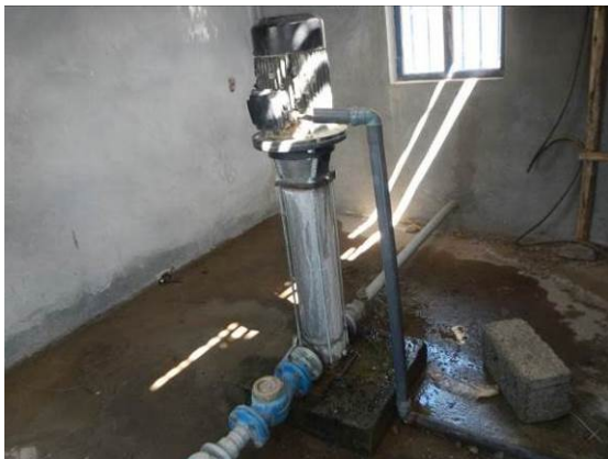
Figure 1-45 Booster pump
