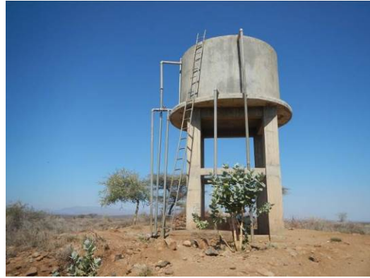
Figure 1-34 Existing elevated tank
