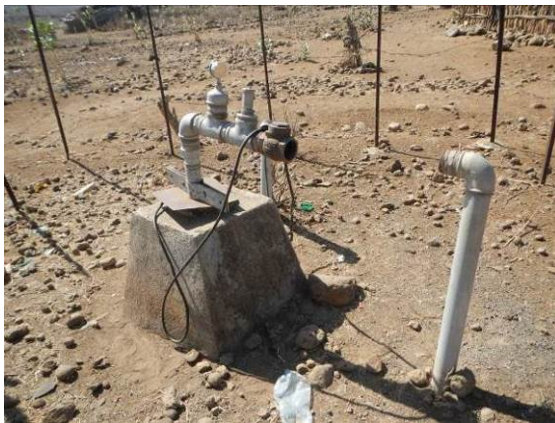
Figure 1-32 Production well
