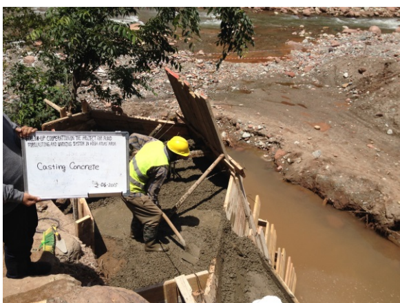
2nd-June Casting Concrete
