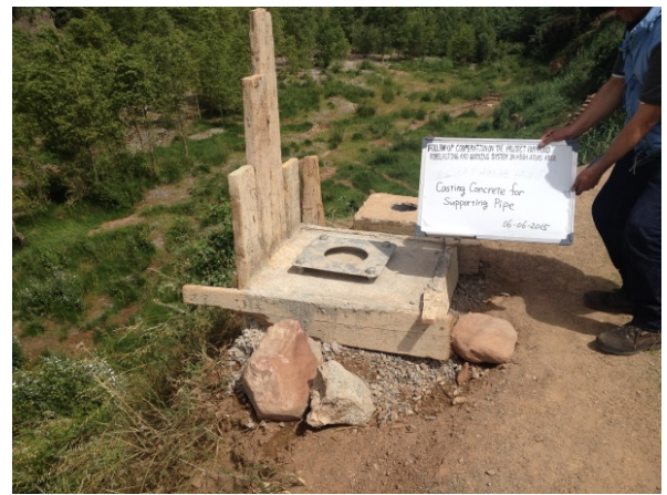
6th June Casting Concrete for steel poles for overhead wiring
