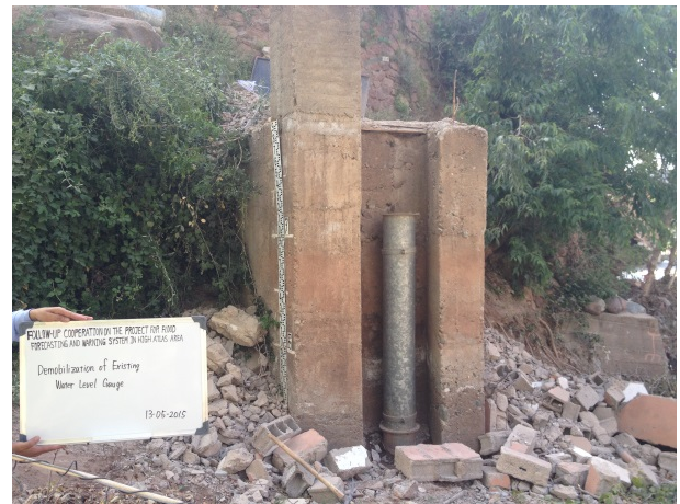
13 th -May Demobilization of Existing Facilities
