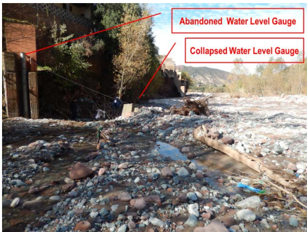
Photo 2.3.1 Location of Reconstruction Site
