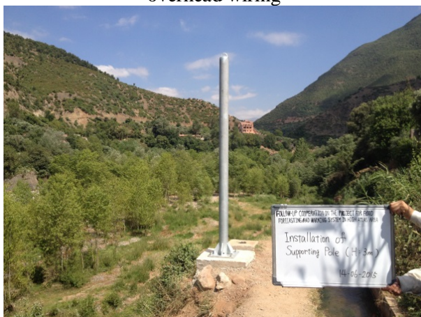
14th June Installation of steel pole (3m) for overhead wiring
