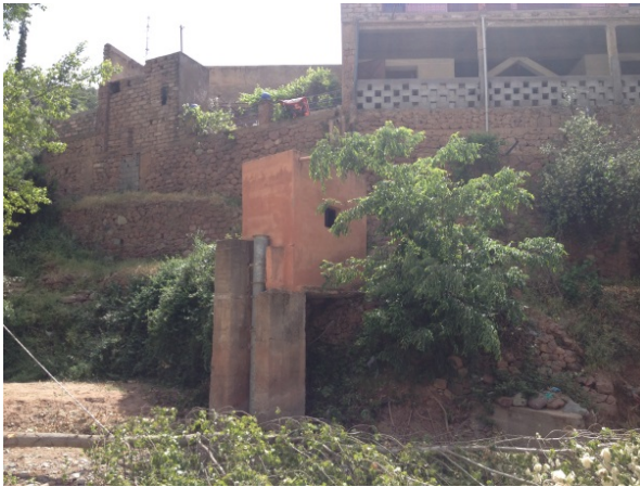
Before Commencement of Work
