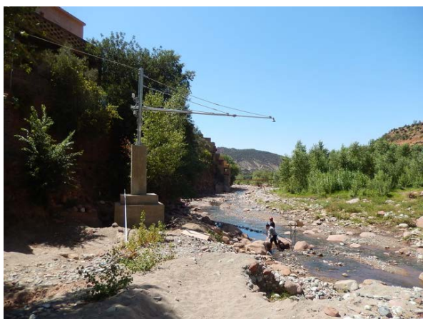
Photo 1.1.1 Water Level Gauge (July 2013)
