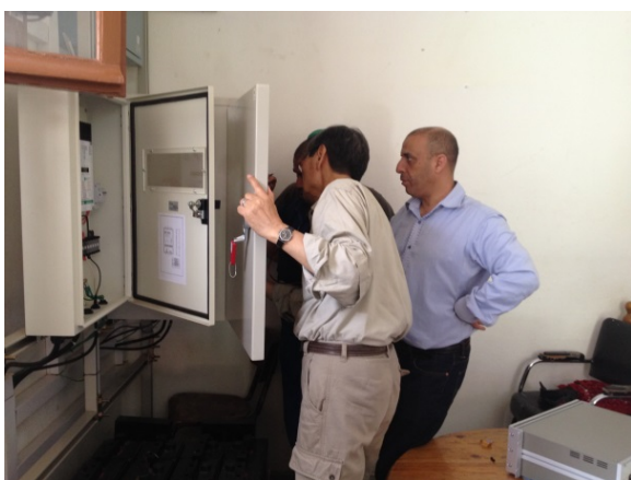
11 th July Installation of main body of water level gauge
