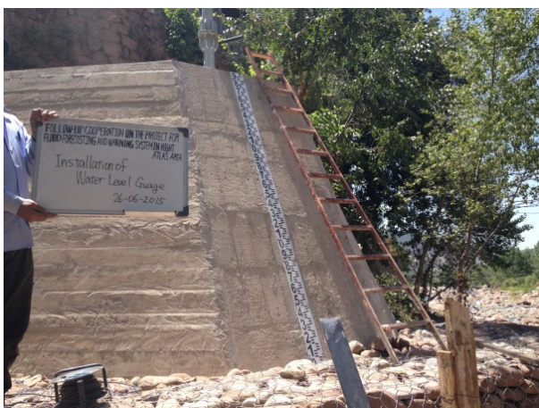
26th-June Installation of water level gauge at concrete structure
