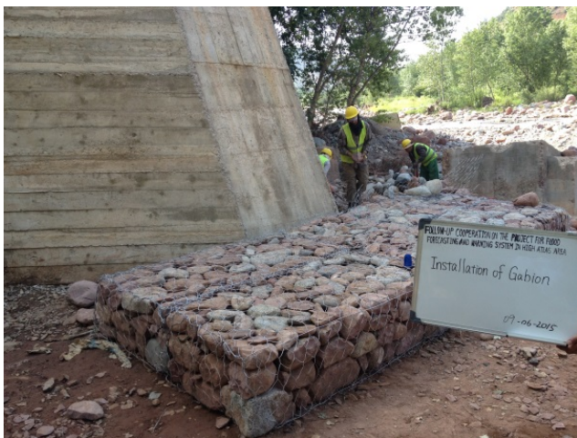
9th-June Installation of Gabion
