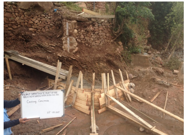
25th-May Casting Concrete
