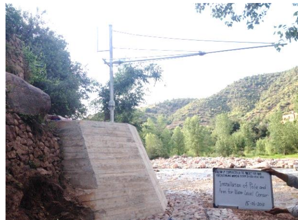
15th-June Installation of arm and pole for water level gauge
