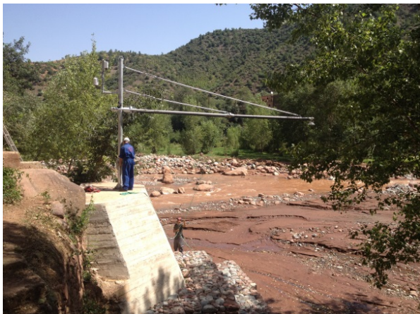
9 th July Installation of transducer and thermometer transmitter
