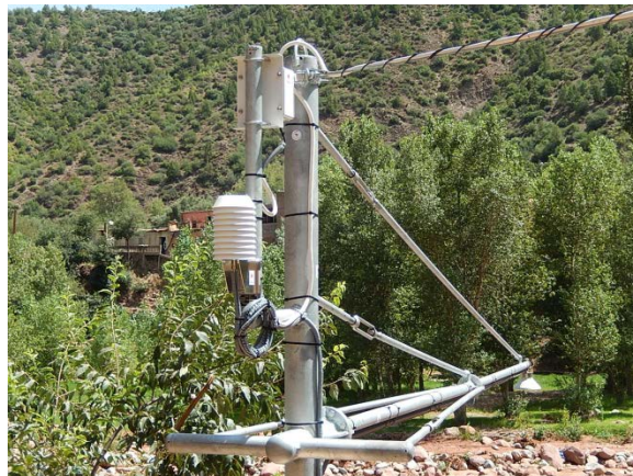
11 th July Completion of installation of transducer and thermometer transmitter
