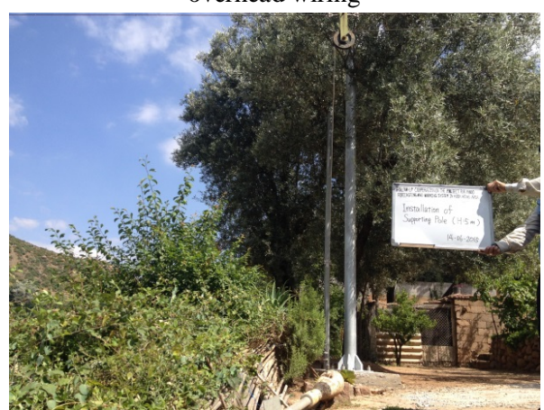
14th June Installation of steel pole (5m) for overhead wiring
