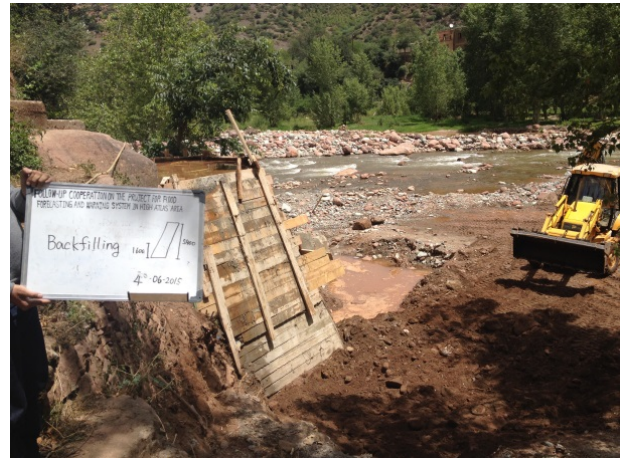
4 th -June Backfilling
