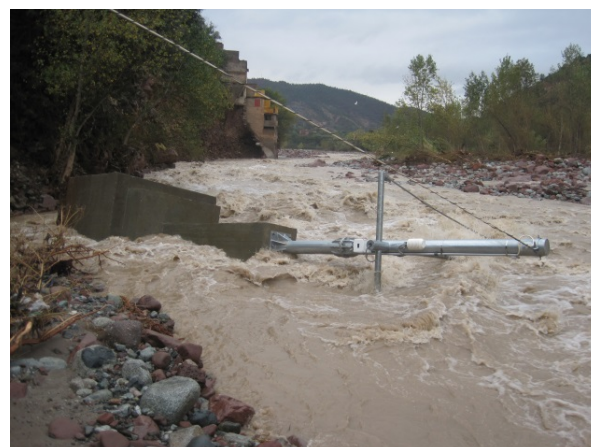
Photo 1.1.2 Collapsed Water Level Gauge (Nov. 2014)
