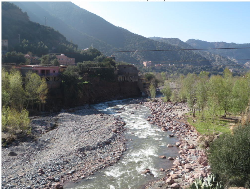
panoramic view 1 (before commencement of work)
