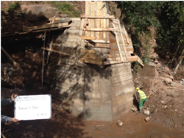
4 th -June Removal of Frame (under part)
