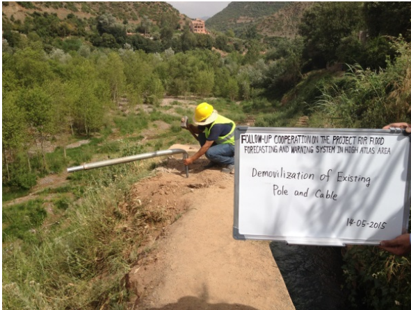
14th May Removal of the destroyed steel poles for overhead wiring
