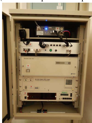
11 th July Completion of installation of main body of water level gauge
