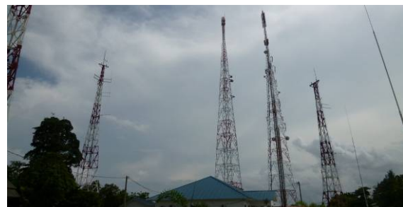
(2) : Steel Towers beside VTS Center
