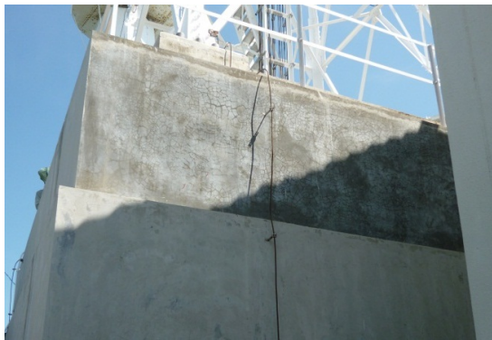
(1) Earth Terminal at Steel Tower Leg
