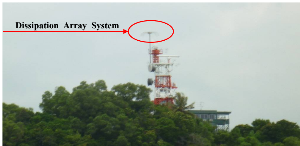
Photo 2-10 Dissipation Array System (made by Hitachi) used in MPA Singapore
