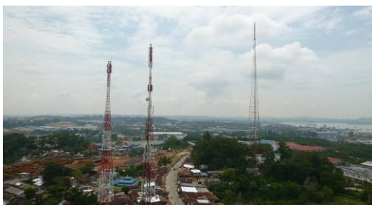
(1) : Steel Towers near VTS Center
