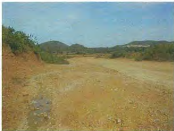
Photo5: Water deterioration risk at a Candidate Borrowing Pit
