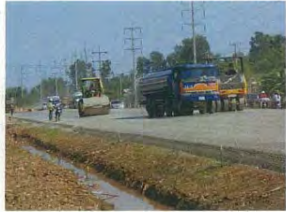
Photo4: Sprinkling at a Construction Site
