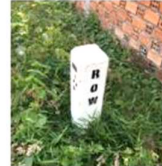
ROW pole for boundary demarcation
