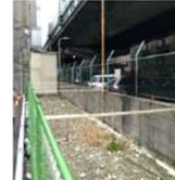
Fencing for preventing encroachment
