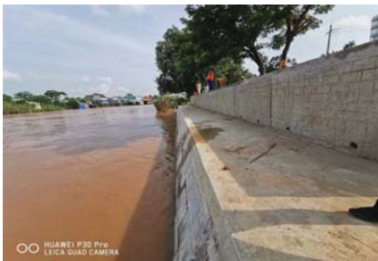
River bank protection at Chrey Thom Village
