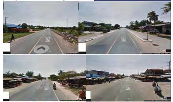
NR.3 After Rehabilitation
