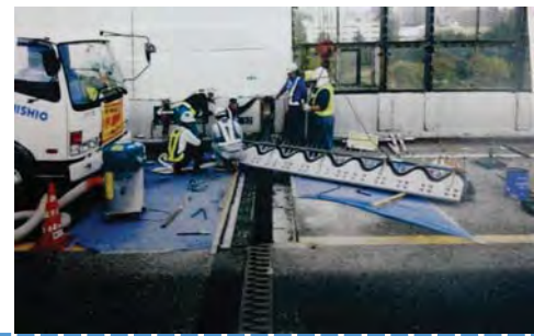
Capacity Enhancement on Environmental and Social Considerations in Implementing Agency in Road Sector
