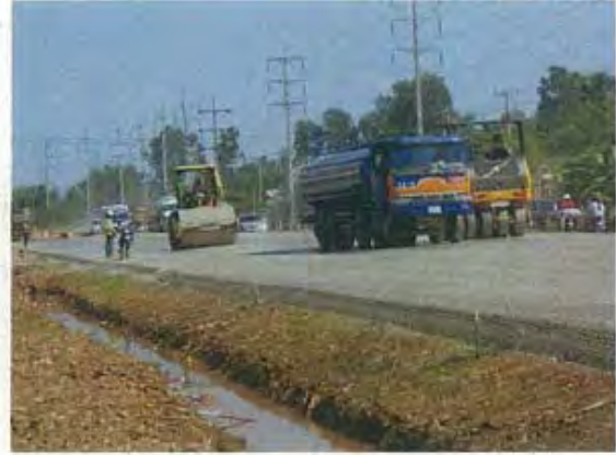
Photo4: Sprinkling at a Construction Site
