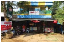
Facility Extended to ROW from Permanent Structure
