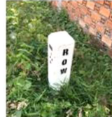
ROW pole for boundary demarcation
