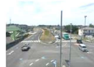
Construction from outside of ROW with service road as the border of ROW
