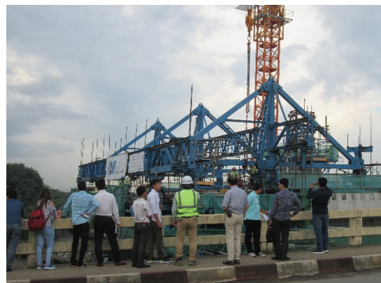
Site visit at New Thaketa Bridge construction site
