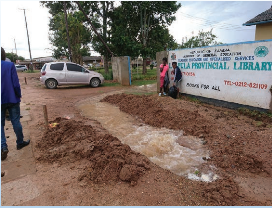
Leakage from Distribution Pipes
