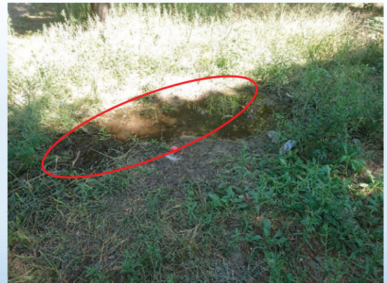
Leakage from Distribution Pipes
