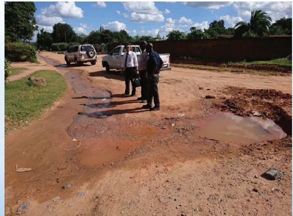
Leakage from Distribution Pipes
