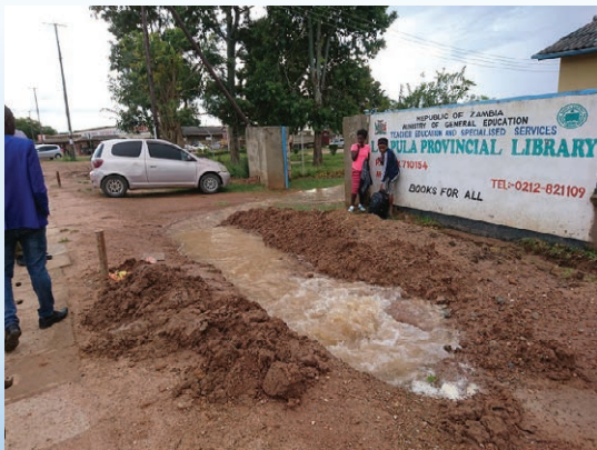
Leakage from Distribution Pipes
