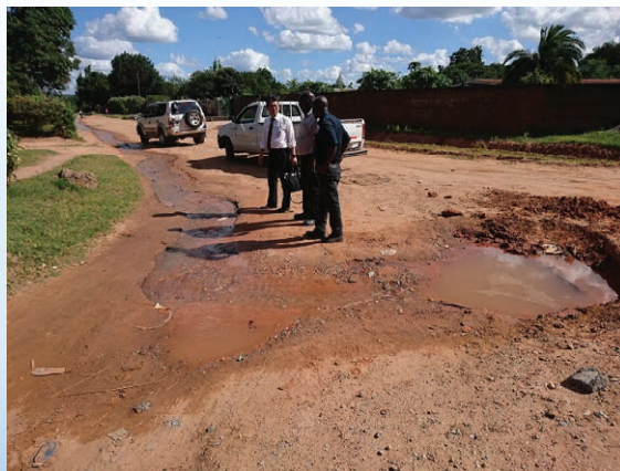
Leakage from Distribution Pipes
