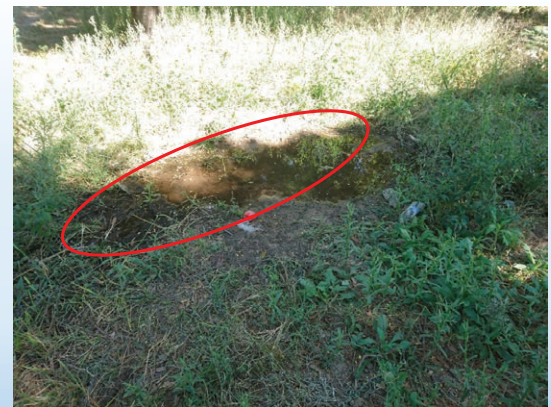
Leakage from Distribution Pipes
