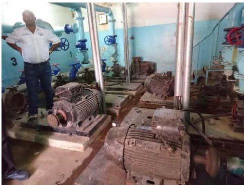
Distribution Plant WWSC (Oct.2018)
