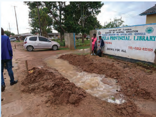
Leakage from Distribution Pipes
