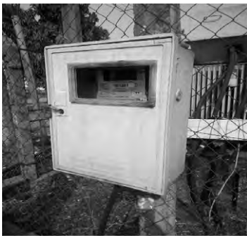
Existing Transformer 1*2.5MVA 33/11kv
