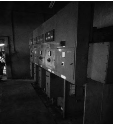
Existing Transformer 7.5MVA 33/11kv
