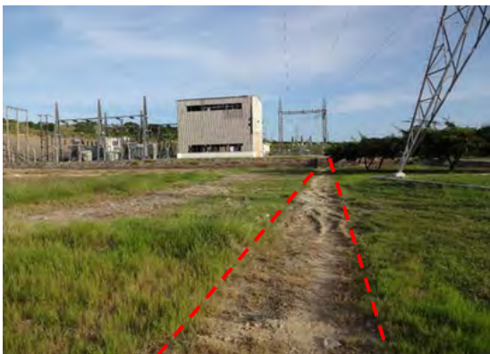
Photograph 2-7 Existing Cable Trench (1)
