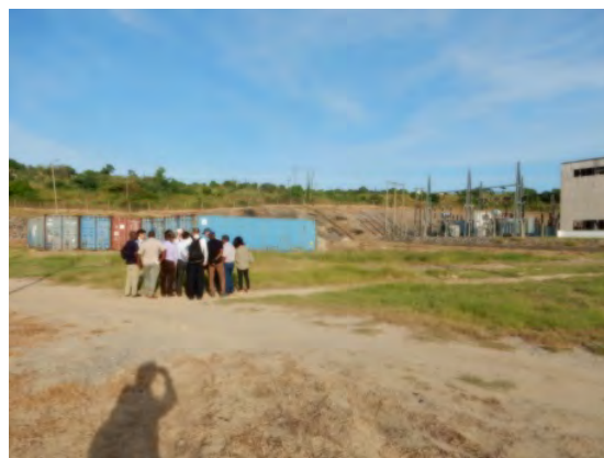
Photograph-2 Proposed site for emergency Nacala power plant; taken in direction of existing switchgear
