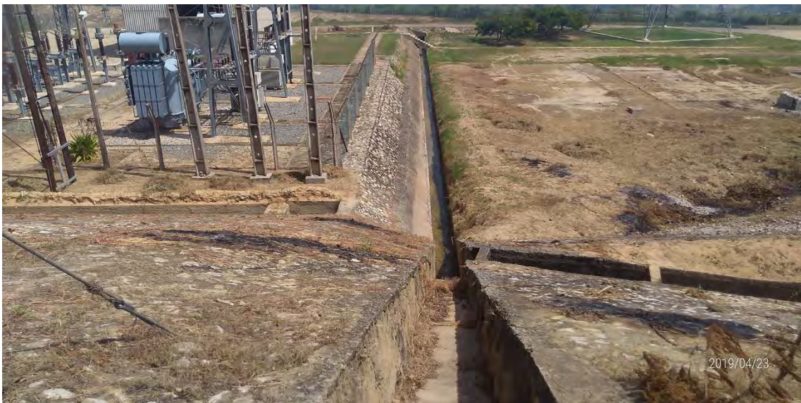
Photo 10: Drainage channel at north side of the substation equipment
