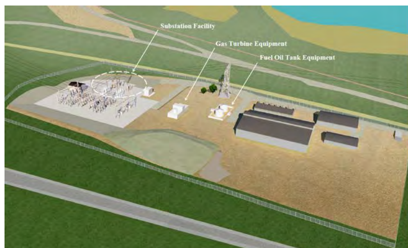
Figure 2-1 Aerial view of Nacala Emergency Power Plant
