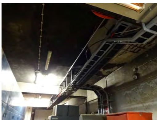
Photograph 2-4 Existing Cable Route
