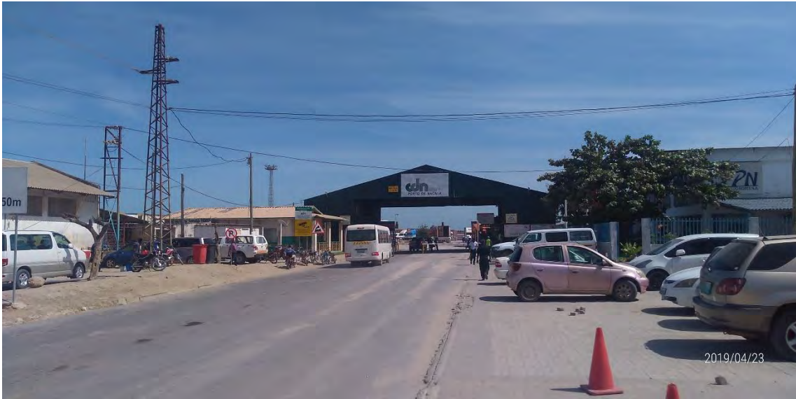
Nacala Port Entrance Gate (height limit 5.5m)
