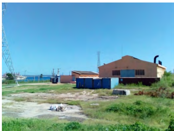
Photograph-1 Proposed site for emergency Nacala power plant; taken in direction of Nacala Bay
