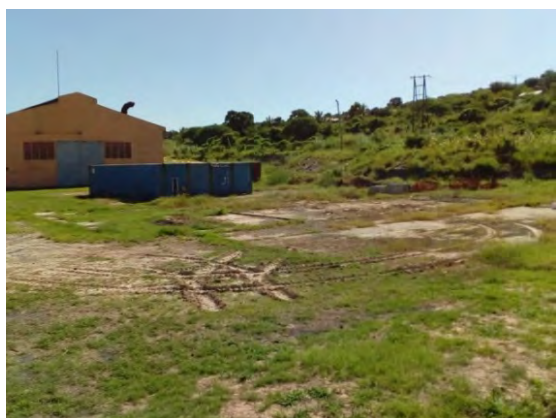
Photograph-3 Proposed site for emergency Nacala power plant; taken in direction of existing Nacala substation control building
