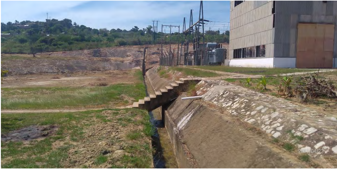
Photo 5: Drainage channel at north side of the existing substation equipment
