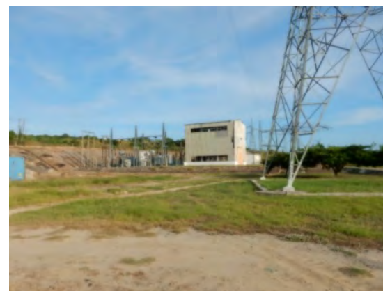
Photograph-6 Proposed site for emergency Nacala power plant; taken in direction of existing pylon and existing substation maintenance building
