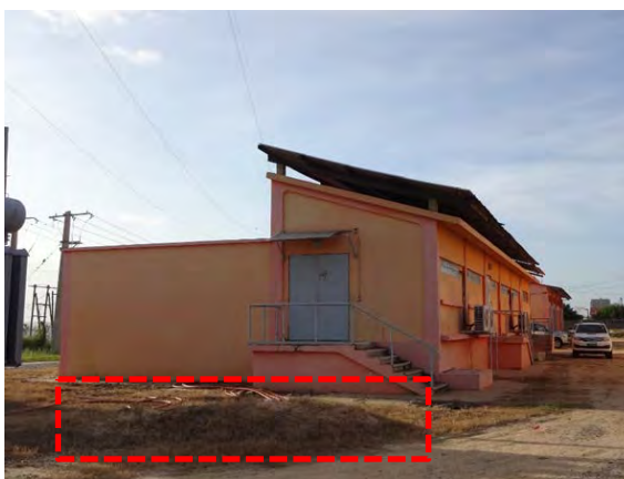
Photograph 2-3 Location where the 33 kV Switchgear Building can be Installed
