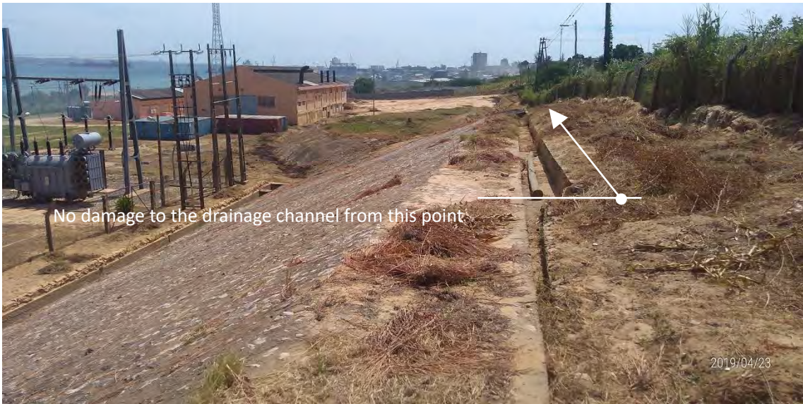
Photo 9: Drainage channel at eastern edge of the substation
