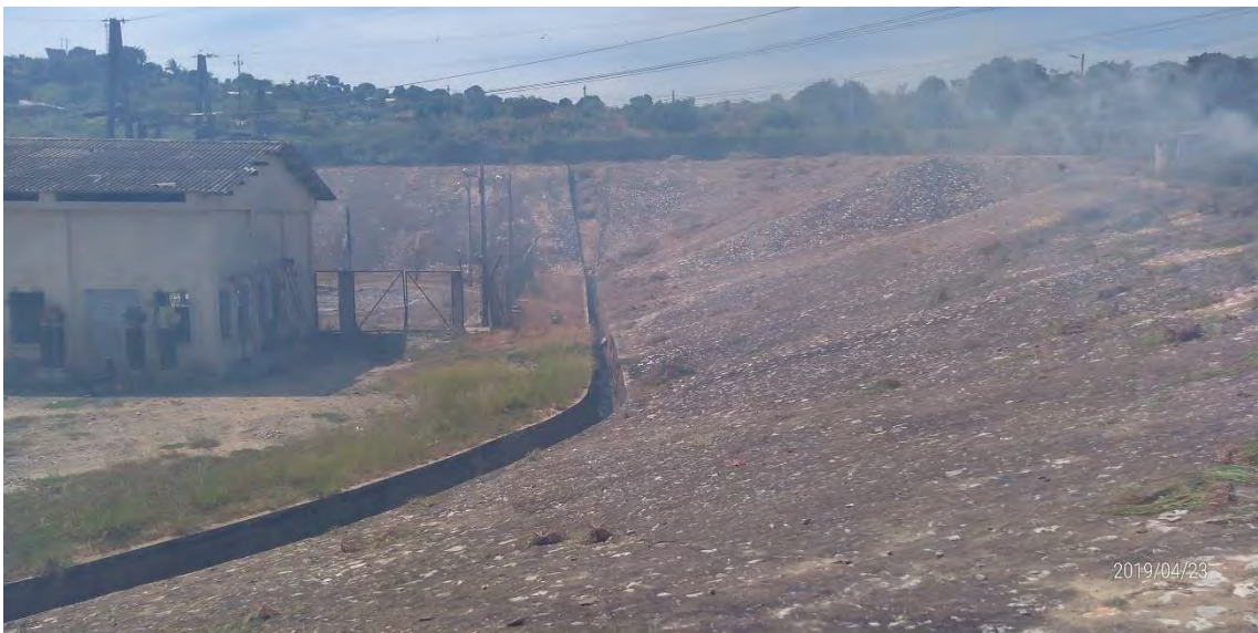
Photo 6: Drainage channel at south side of the existing substation equipment
