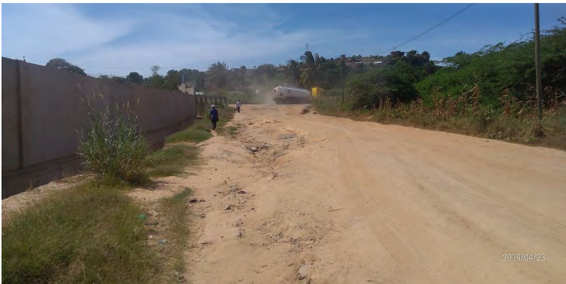
Unpaved road at north side of the site 2 (surface is uneven and rough)
