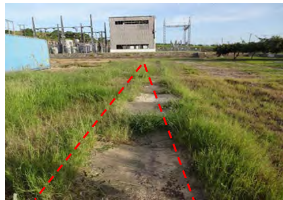
Photograph 2-6 Existing Cable Trench (2)
