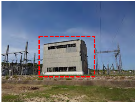
Photograph 2-5 Existing Transformer Maintenance Building
