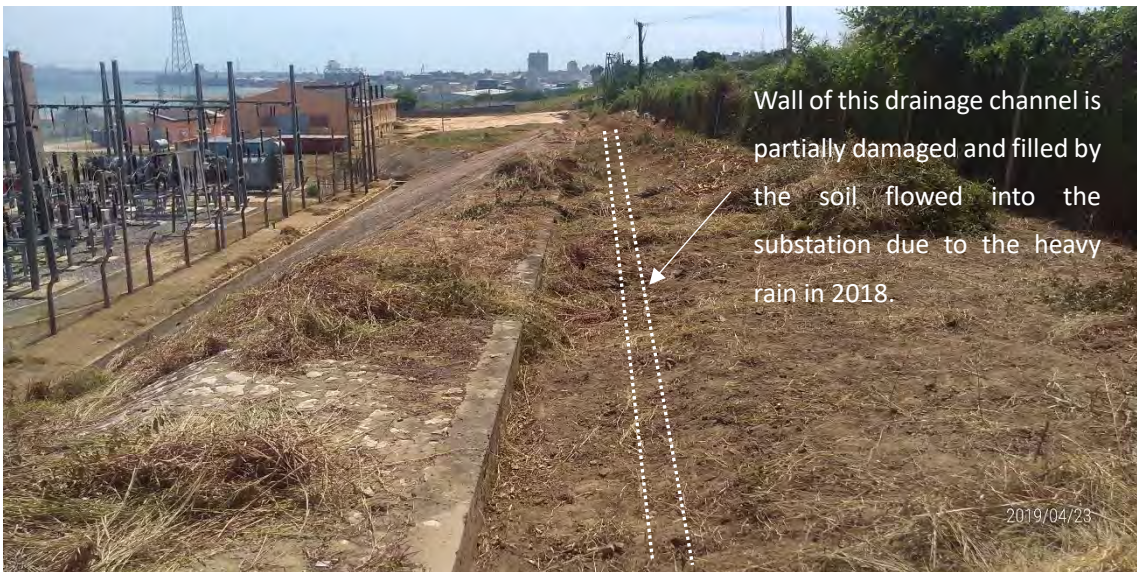
Photo 8: Drainage channel at eastern edge of the substation
