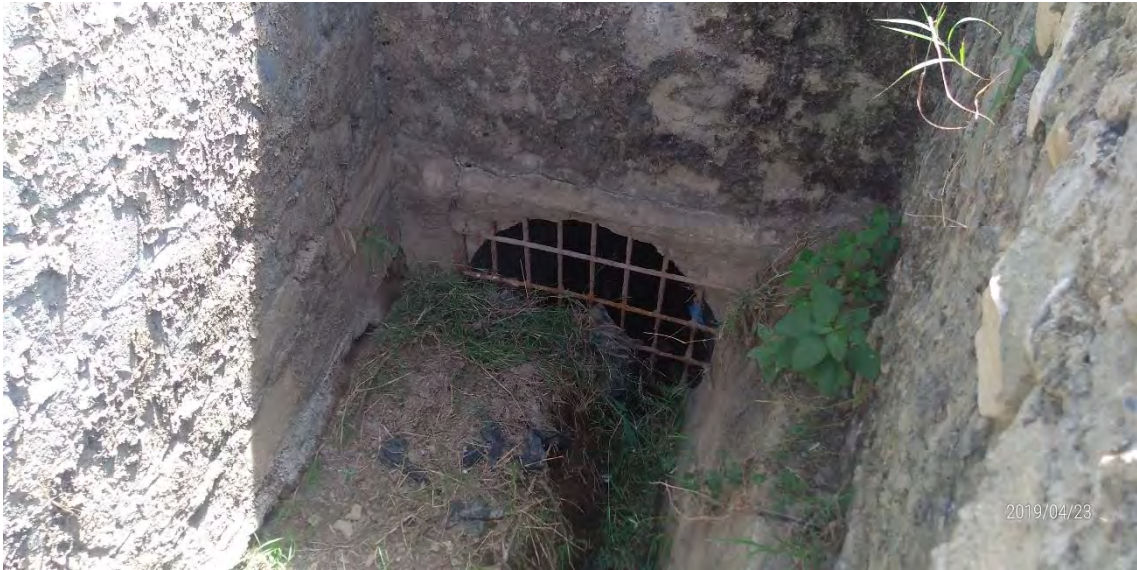
Photo 3: Drainage pipe at west side of the substation
