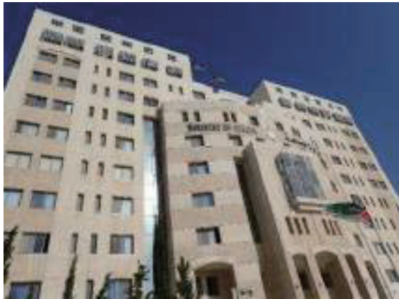
(April 2016) Ministry of Health (MOH) Headquarters
