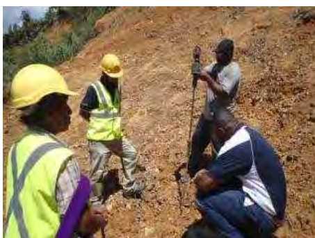
Dynamic Cone Penetration Test (DCP) at Ch. 1+300 is carried out in order to find the cohesion of the soil.
