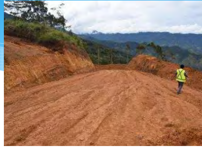
Type 'D' Excavation (slope cutting) is completed from Ch.4+800 to Ch.6+200
