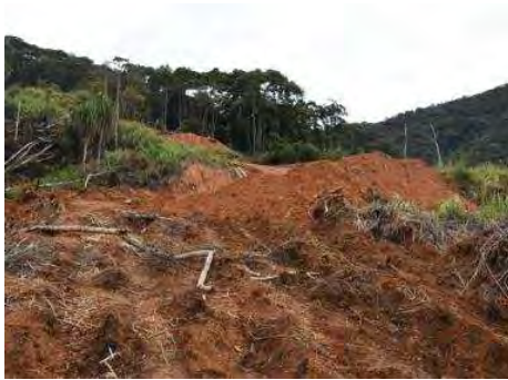
Laying of capping layer from Ch.4+400 to Ch.6+200.
