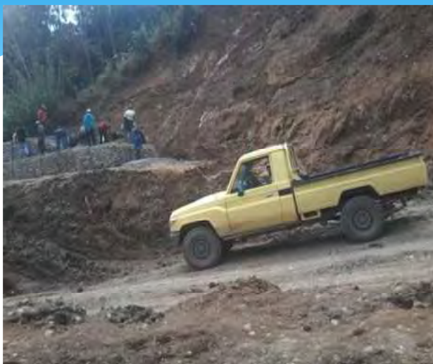
Clearing, loading and excavation for gabion works at Ch. 1+00
