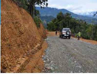
Clearing/Grubbing is completed from Ch.4+900 to Ch.6+300.
