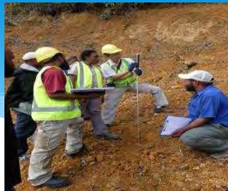
Penetration Resistance Test by Soil Strength Probe at Ch. 1+300.
