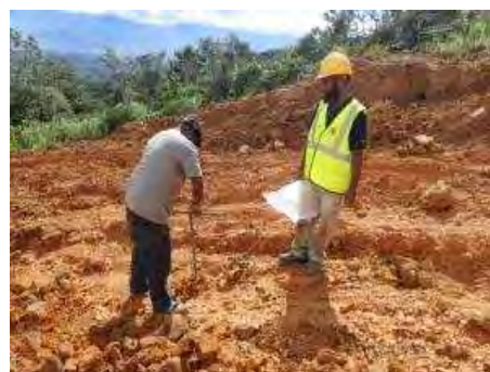
Sample collection for moisture content test at Ch. 6+200
