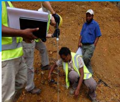
Vane Cone Shearing Test Soil Strength Probe at Ch. 1+300.
