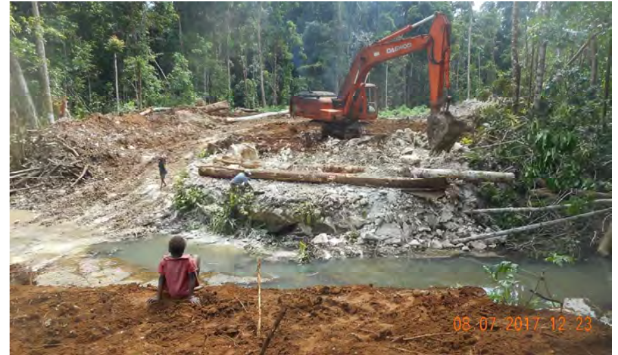
Log Bridge abutment construction – Vil Creek
