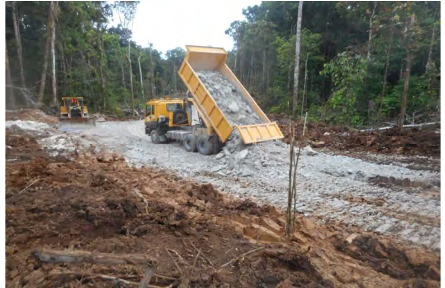
Sub Base material - Graveling Works at CH: 14.5km
