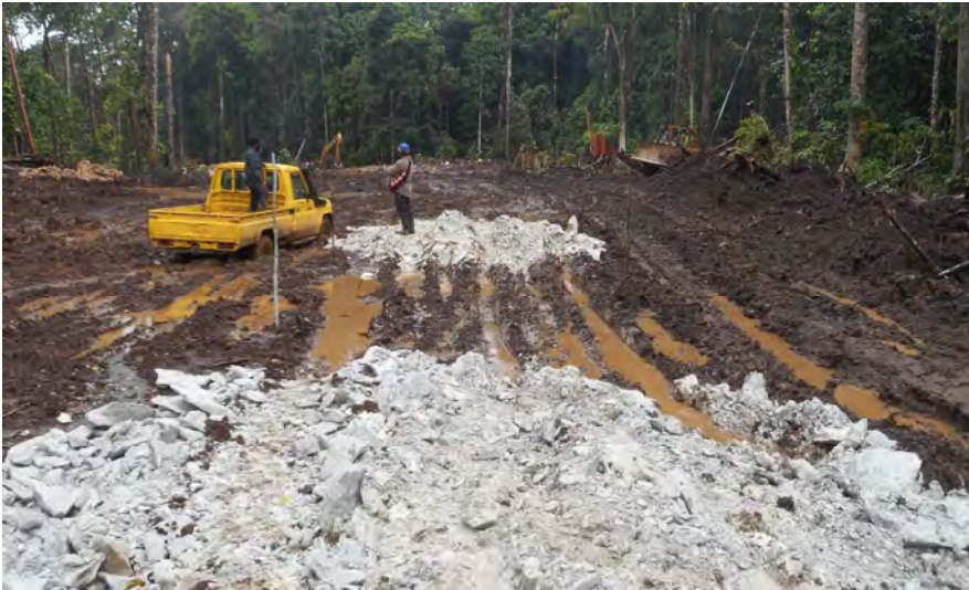
Wet days on project site
