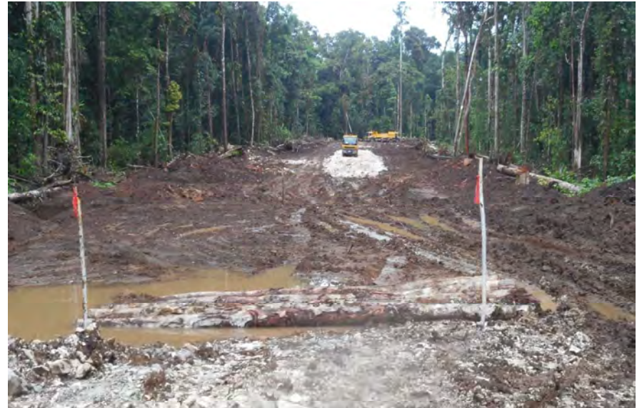
Daily activity (Gravelling) suspend due to rain
