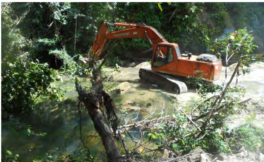
Wet crossing at Vol river – During construction
