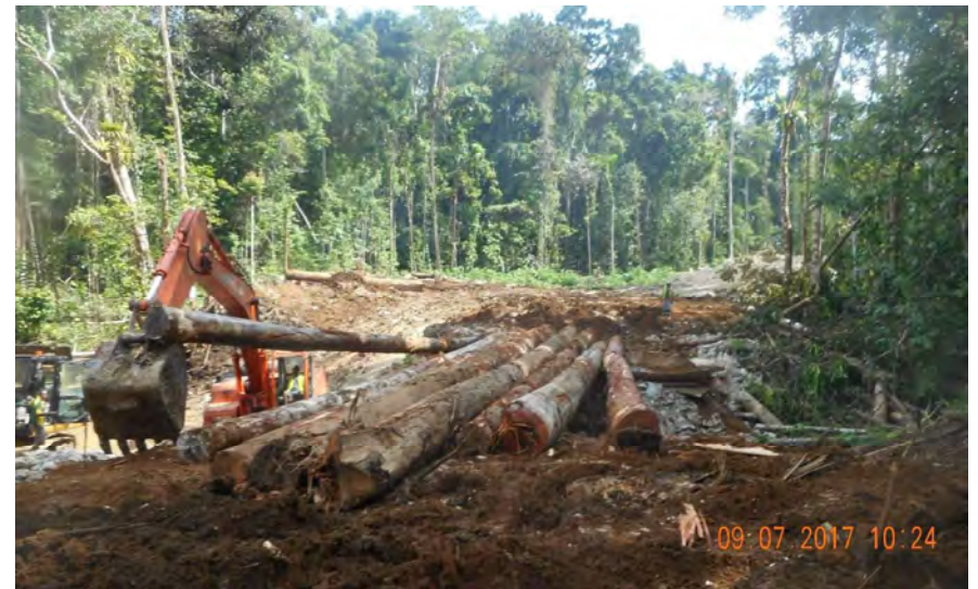
Log Bridge construction – Vil Creek
