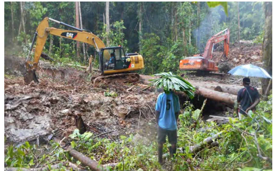
Tavurlasi Log bridge construction
