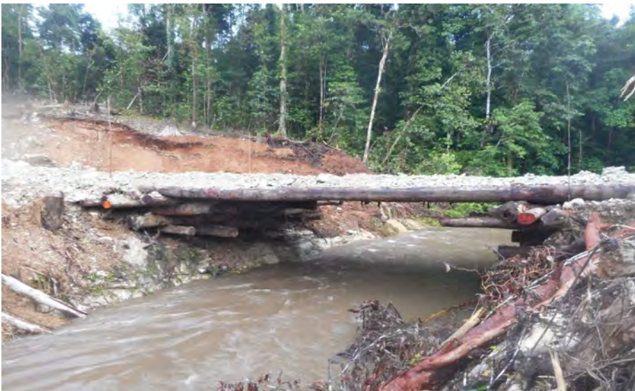
Completed - Akress temporary Log Bridge access
