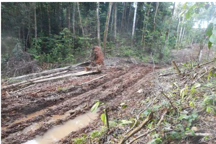
Trees felling CH: 15.5km to CH: 18.0km
