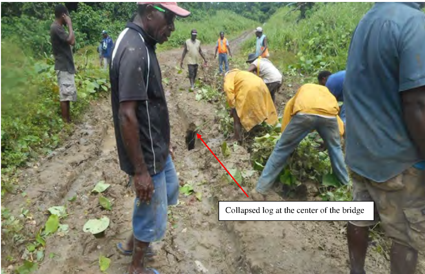
Workmen repairing part of the Collapsed temporary Log Bridge excess about 10km from Silovuti Junction and 30km to start of Project site.
