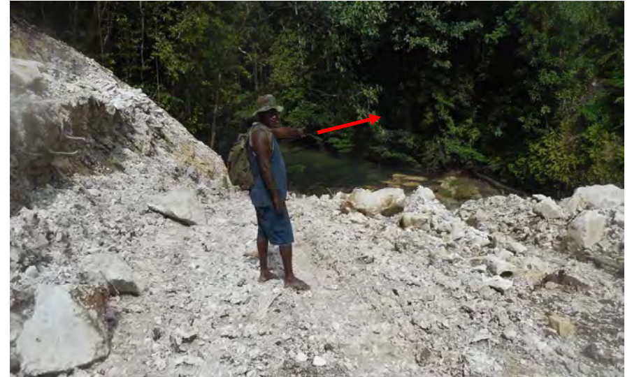
Vol River – Wet crossing (Photo before)
