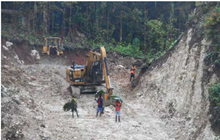
Clearing mud and gravel patching by Dozer & Excavator during wet weather
