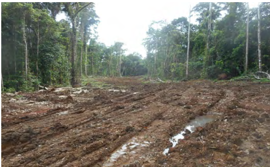
Clearing and Grubbing works CH: 14.5km to CH: 15.5km
