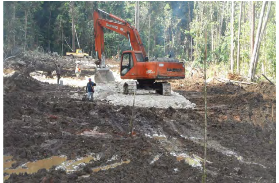
No option!! But to use Excavator and Dozer for gravelling work during wet days.
