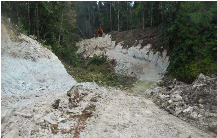
Vol River wet crossing – Kimbe approach (photo after)
