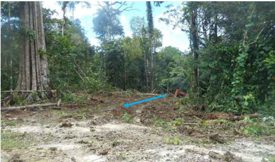
Road connected - Vol river Kandrian approach. (Propose Road connection alignment) Photo after
