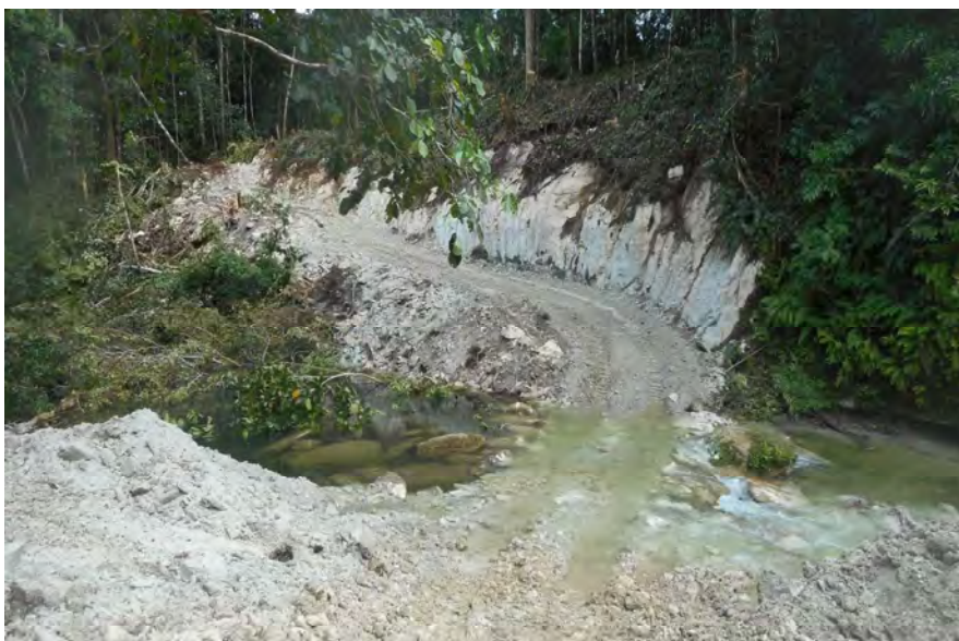
Wet crossing at Vol river after construction
