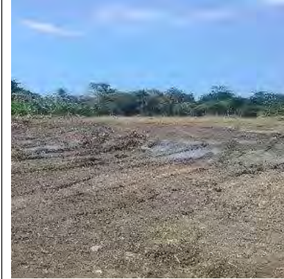
Clearing & Grubbing Works
