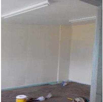
Office completed and painting in progress
