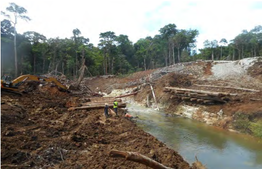
Akress River construction phase
