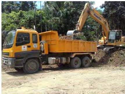
Clearing Works CH 1+800
