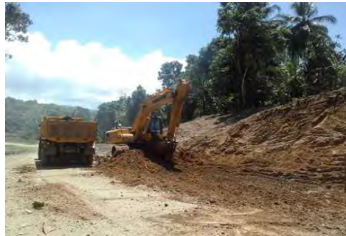
Excavation Works CH 1+950
