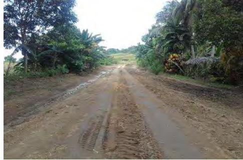
Clearing Works CH 0+500
