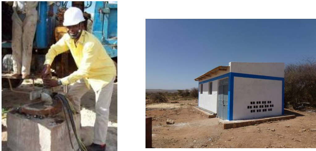
Figure 2.2: Installation of Riser Pipe (left) and Generator House Completed (right).
