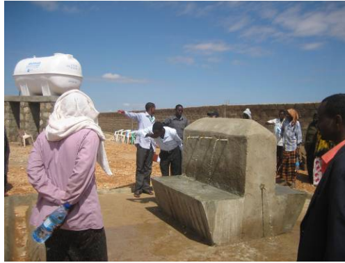
Figure 2.5: Water Supply Point (Construction completed at Kabribeyah Town)
