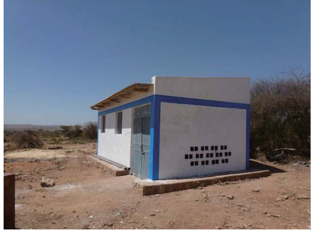
Construction works of water supply facilities (1)
