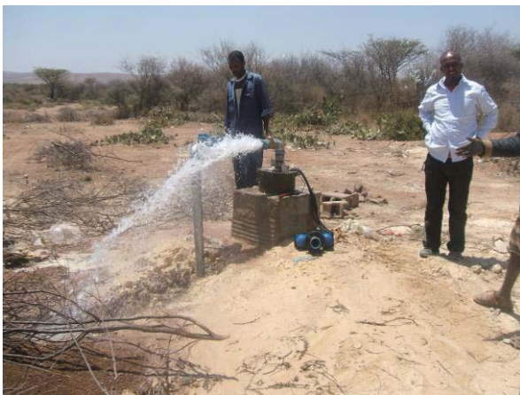
Pre-operation test of constructed wells
