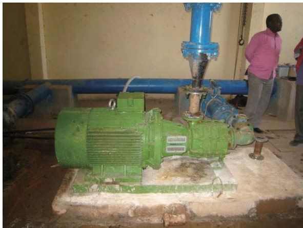
Construction works of water supply facilities (2)
