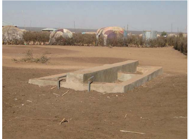
Construction works of water supply facilities (3)
