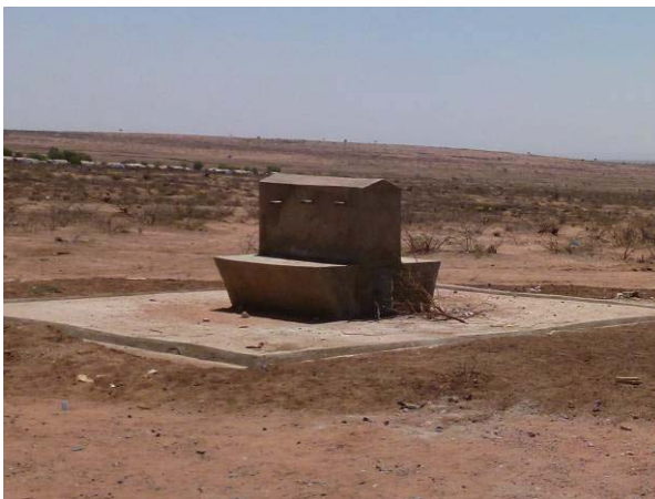
Construction works of water supply facilities (4)
