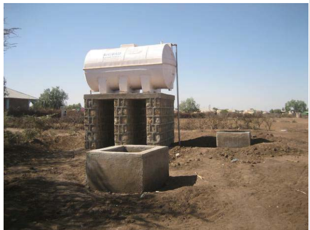
Construction works of water supply facilities (5)
