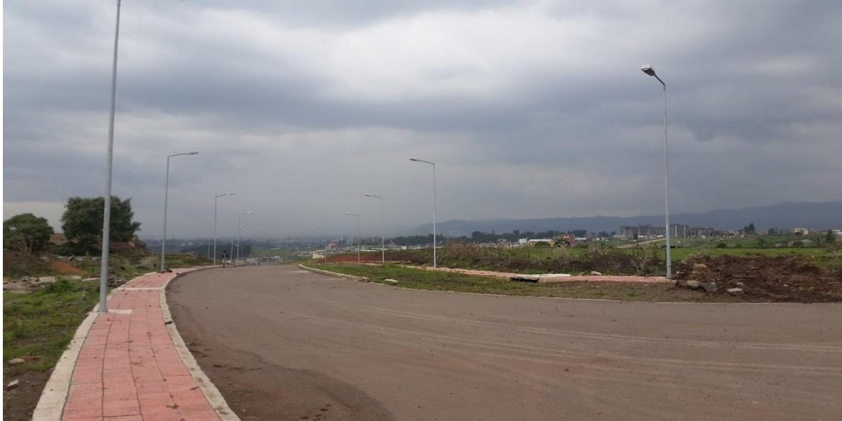
Picture 4: Existing Street Lights
