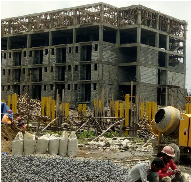
Picture 2: One of the Dormitory's Under Construction
